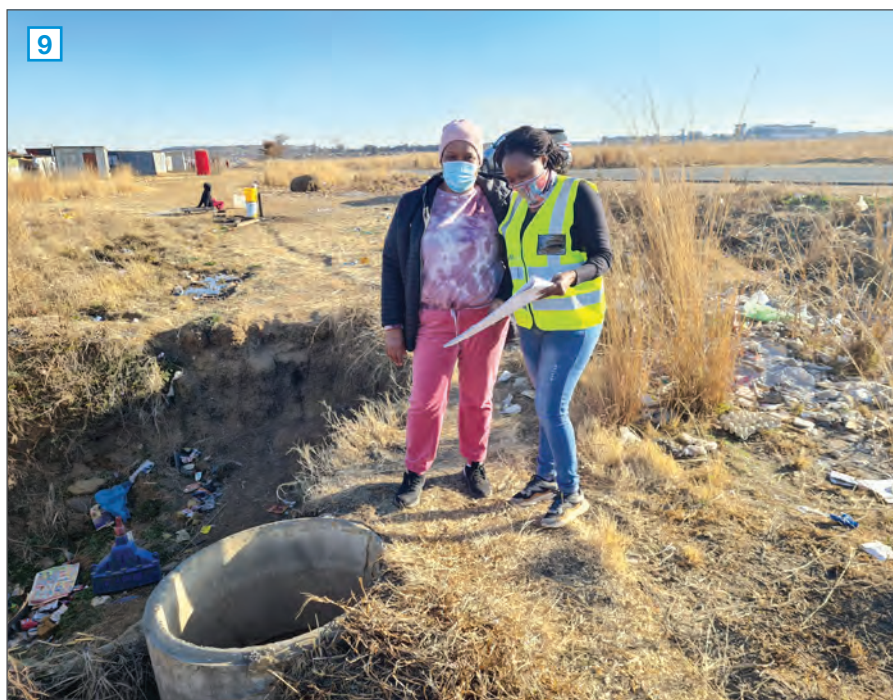
Figure 9: Phathi Masimirembwa reviewing alignment for the proposed Evaton reservoir to Dadaville bulk water supply pipeline for Emfuleni Municipality
