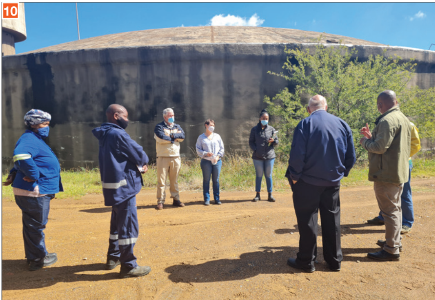
Figure 10: SAICE-PDP experts, Metsioa Lekwa team, at the Vanderbiljpark reservoirs discussing how to isolate one of the 27 ML reservoirs with a non-functional isolation valve to enable repair of the valve
